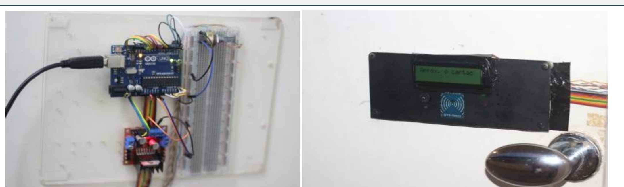
Access Control System Module (ACS)
